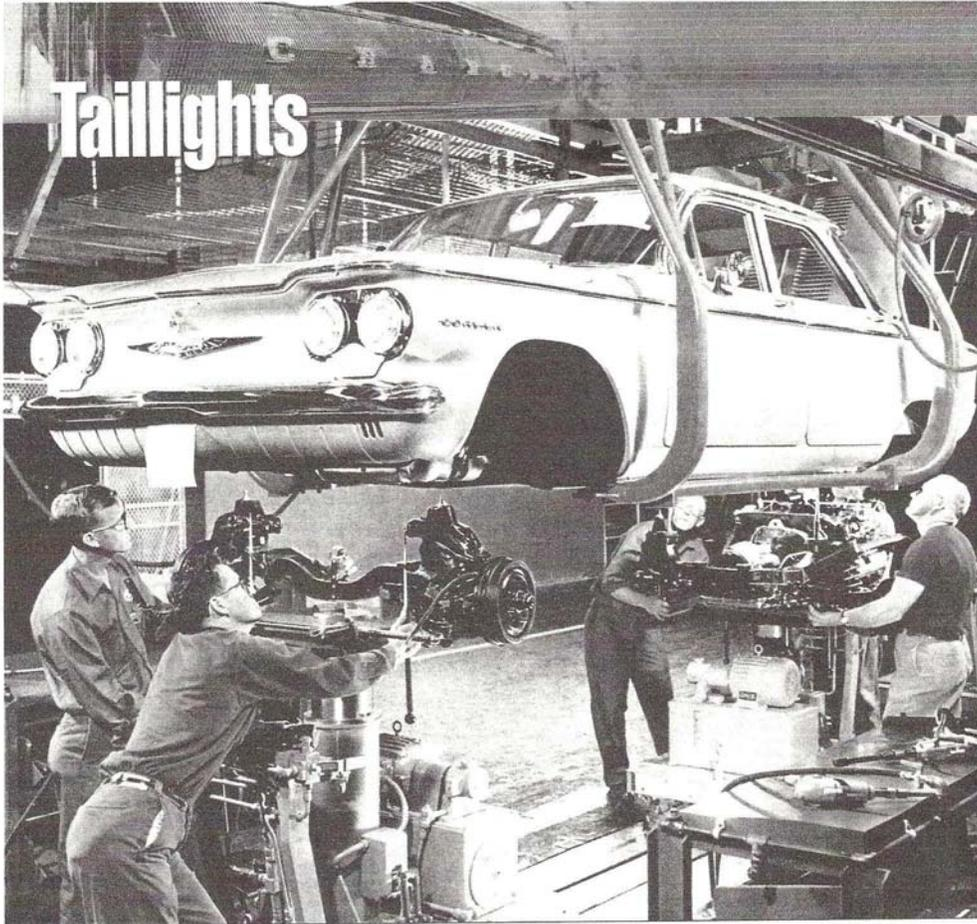
**BY BOB STEVENS** ■ CHEVROLET'S WILLOW RUN ASSEMBLY PLANT WAS A MODERN MARVEL OF HIGH-TECH PRODUCTION PROCESSES WHEN IT OPENED IN 1959. YET IT WAS UNLIKE ANY OTHER AUTOMOTIVE PRODUCTION PLANT IN THE U.S., A UNIQUE FACILITY DESIGNED AND BUILT EXPRESSLY TO BUILD CHEVROLET'S UNIQUE LITTLE COMPACT CAR, THE REAR-ENGINE, AIR-COOLED, REAR-DRIVE CORVAIR INTRODUCED FOR THE 1960 MODEL YEAR.
