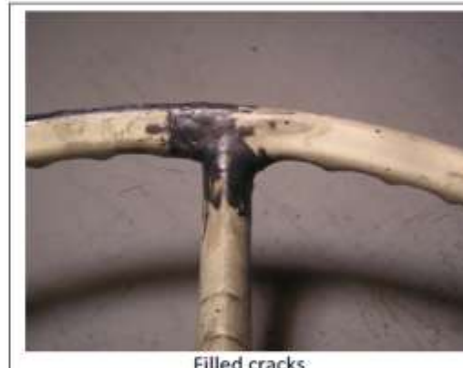
Filled cracks
